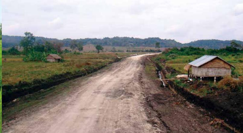
After construction, soil is piled up and compressed to build a reliable road, which is sturdy enough even for large trucks to pass through.
